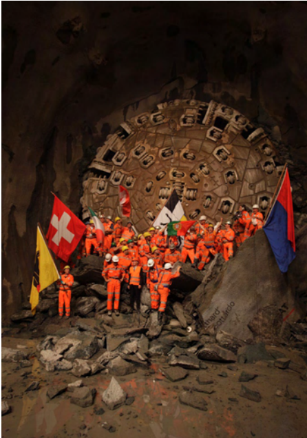
Saint Gotthard Tunnel © AlpTransit Gotthard AG.
